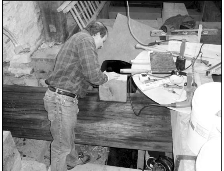
Gus Kiorpes installing the arms of the pit gear.
