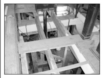
Steve has already begun the next part of the job, that of replacing selected floor joists, the 17-foot beams supporting the main floor that go in both directions from the main beam to pockets in the wall on the west and east sides of the basement. The picture shows sections of the main floor removed so that the crew could gain access to a damaged joist.
