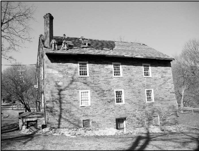
The first section of new shingles is installed.
