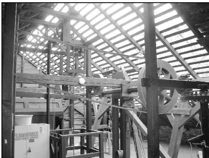
View of the attic with the old shingles removed.
