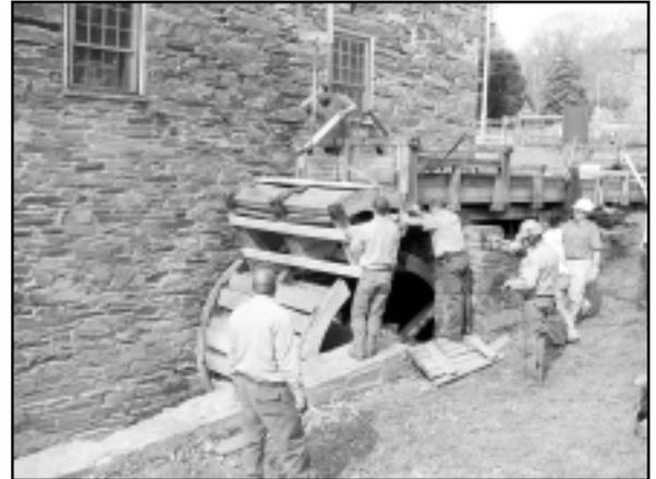
*Lifting out one segment of the water wheel after bracing*
