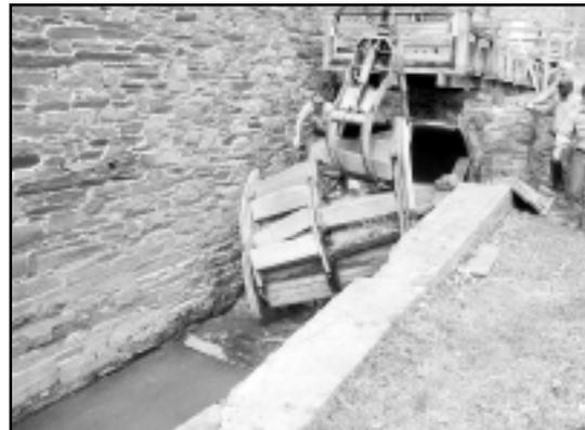
*Lifting out the badly damaged front section of the wheel*
