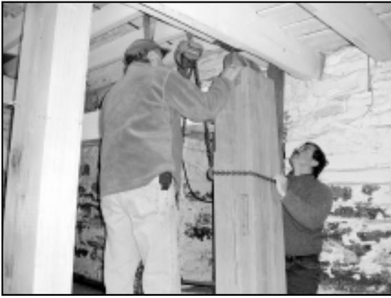
*Installing new right front corner post*
