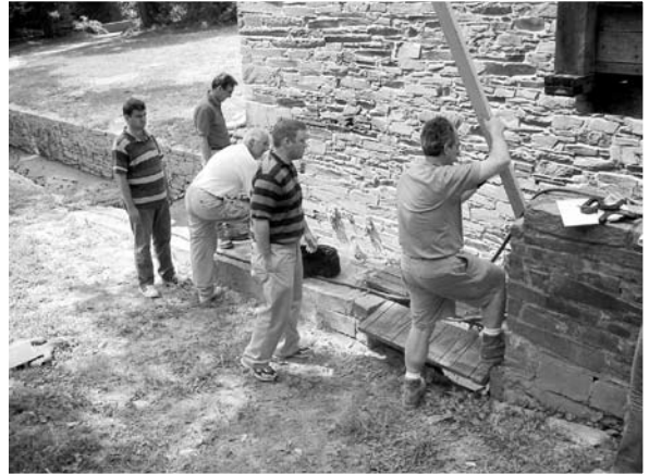
Steve Ortado checks the depth in the tailrace
