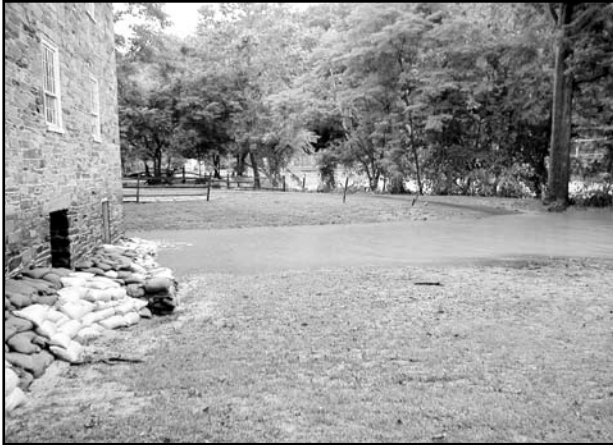
The rear of the mill after the water had receded about six feet
