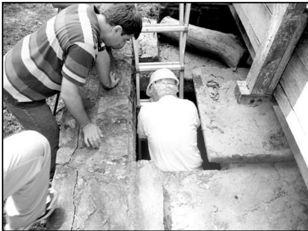
Exploring the old pump pit beneath the flume
