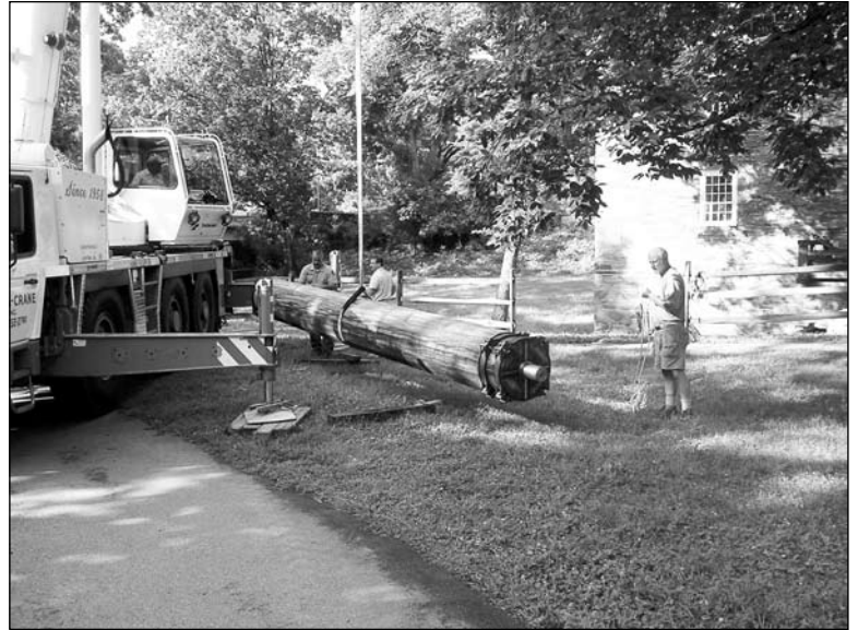
Lifting the shaft
