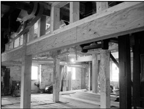
As our first picture shows, the contractor, TMG Corporation, has already excavated a pit where the re-circulating pumps will be installed. These pumps will lift water from below the new water wheel to the head race (yet to be excavated) from whence it will flow down a flume to power the water wheel. Inside the building, TMG has completed installation of additional beams that will strengthen the structure to accommodate much heavier floor loading, as well as heating ducts that will take
