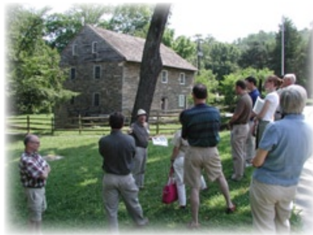
Architect Baird Smith tells Advisory Board members about the condition of the mill building.
